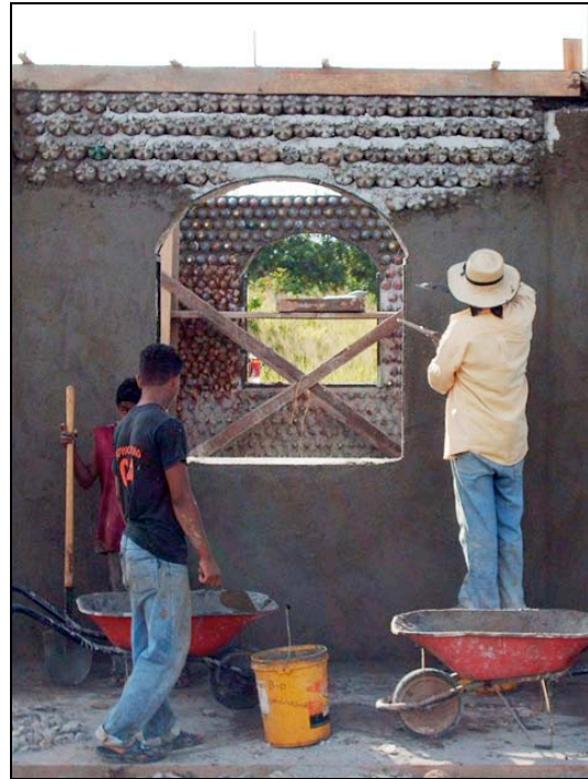
and plaster the walls.
